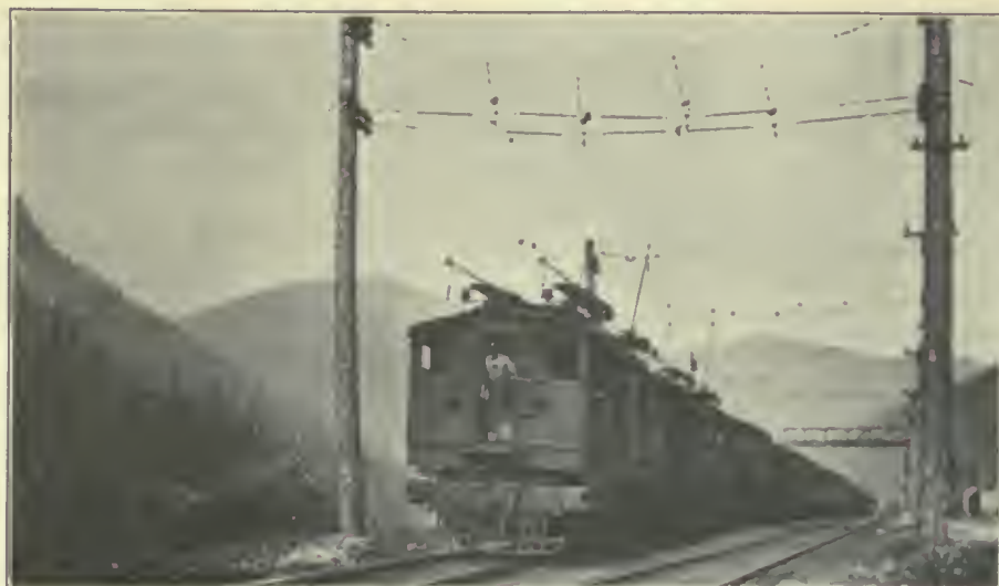
FIG. 524. OVERHEAD CONTACT SYSTEMS. 6,600-Volt Three-Phase Main Line Construction, Great Northern Railway, Cascade Tunnel.
